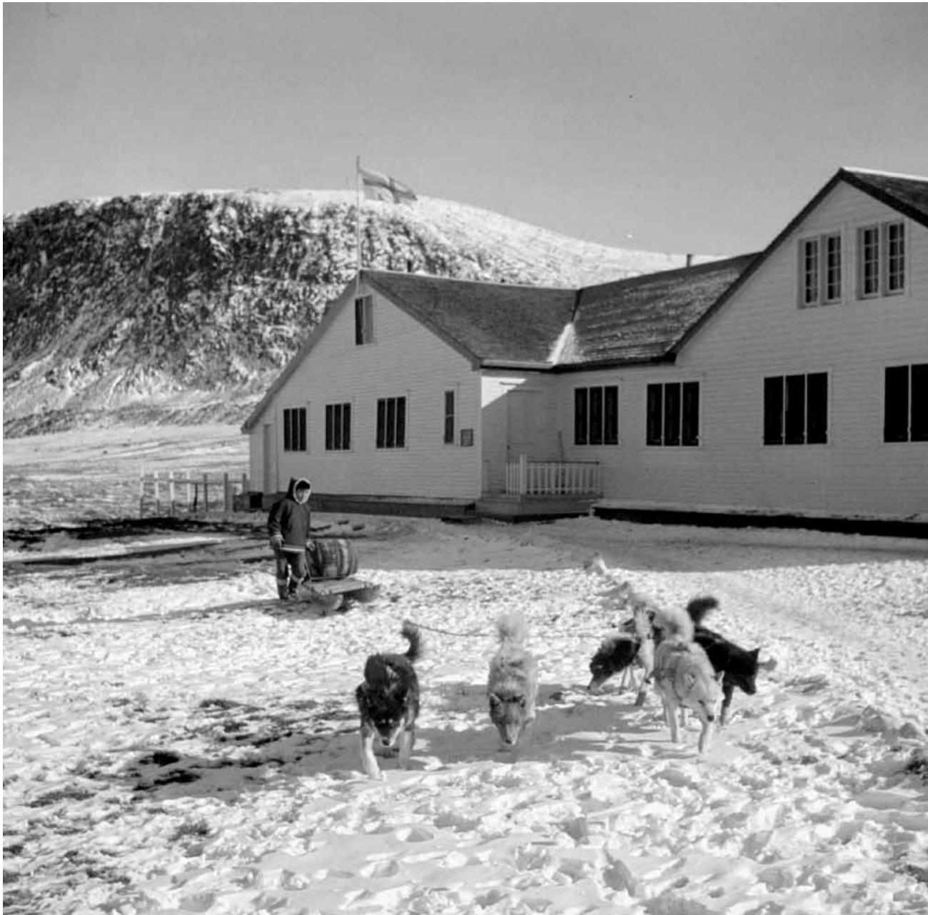
Dog team delivering drinking water to St. Luke's Mission Hospital, August 1946
